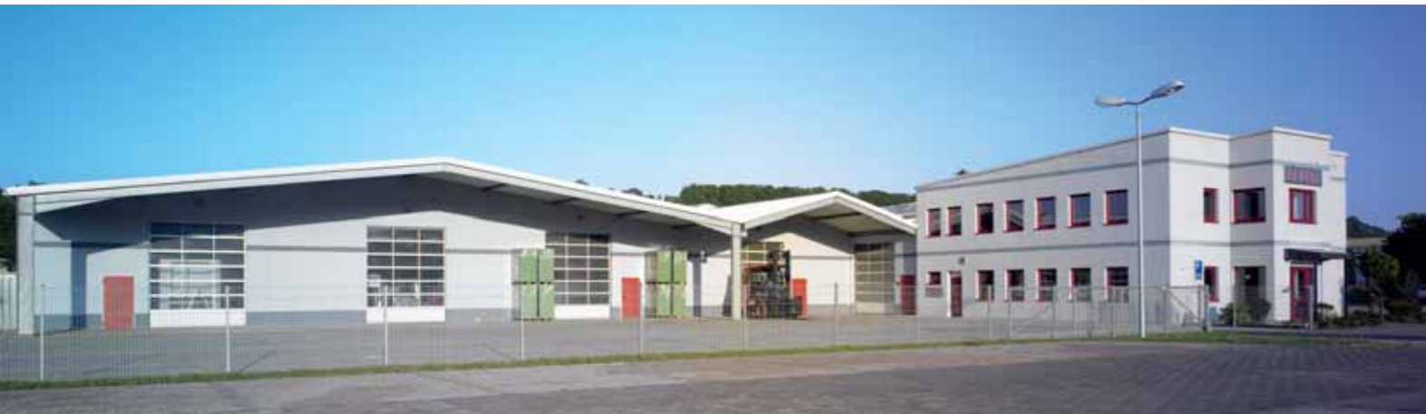
Company headquarters in Konz near Trier
